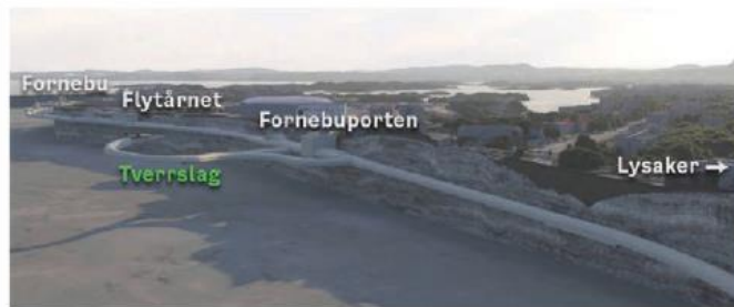
Above: The SiteVision AR tool was used for design on the Lysaker-Fornebu tunnel
