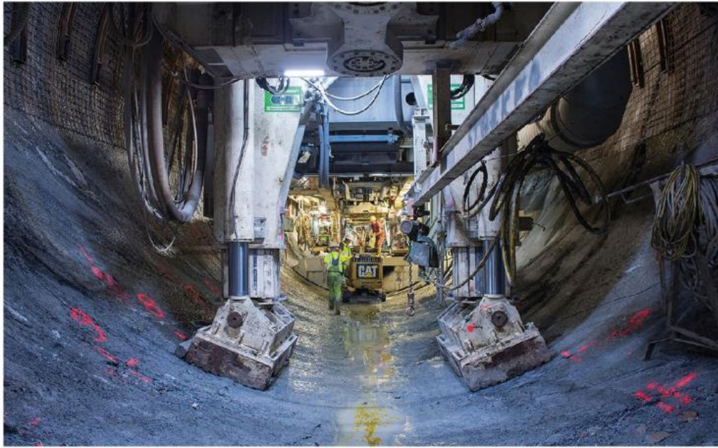
Above: At the Brenner Tunnel, the dataset was built using geological data from the exploratory tunnel IMAGE: BBT
